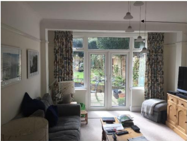
Existing lounge showing as built RSJ and at LHS wall to be removed to open up kitchen
